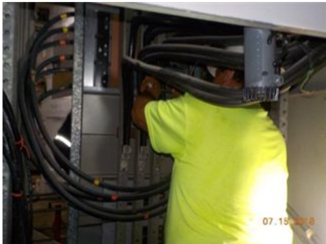
Tighten Terminal Lugs
