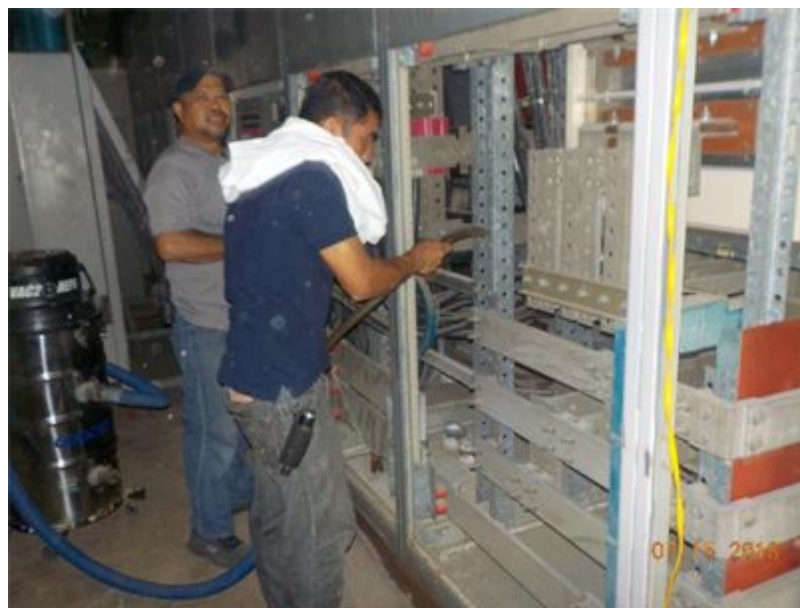
GMH PERSONNEL VACUUMED INSIDE THE COMPARTMENTS AND WIPED BUS BARS AND CABLES
