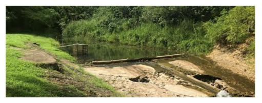
1, The river has become very shallow over the last 10 years at the Intake Area. The buildup of silt should be removed, and the Intake Area restored.
