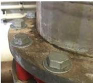
3, Many of the valves were installed using threaded rods that pass through the centers of the lug style connections. These rods are undersized and make it difficult to align the valve / pipework flanges correctly. This in turn causes valves to stick and to leak. The threaded rods should be replaced with the correct sized bolts and washers.
