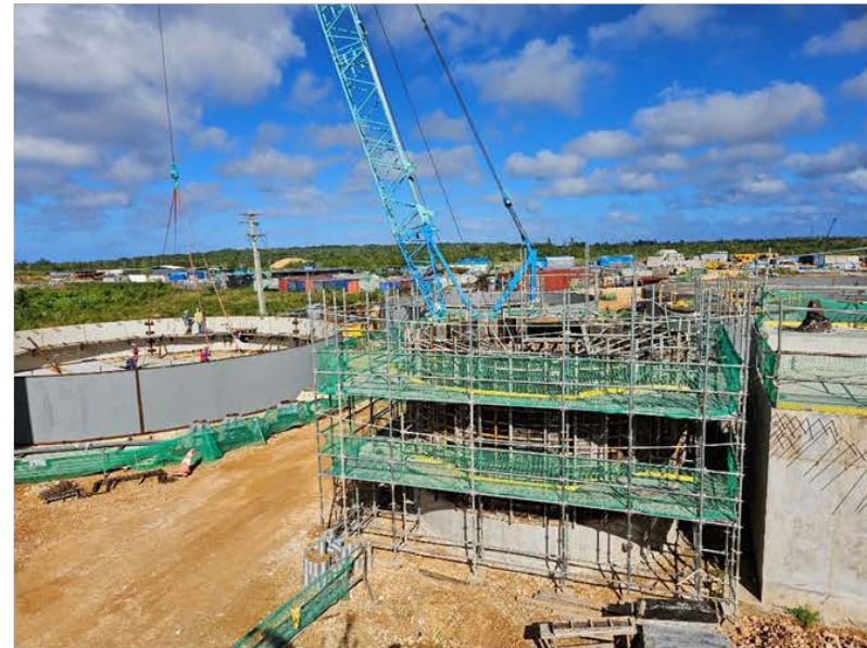
Fire Pump House & Tank – Fire fighting tank installation is ongoing.
