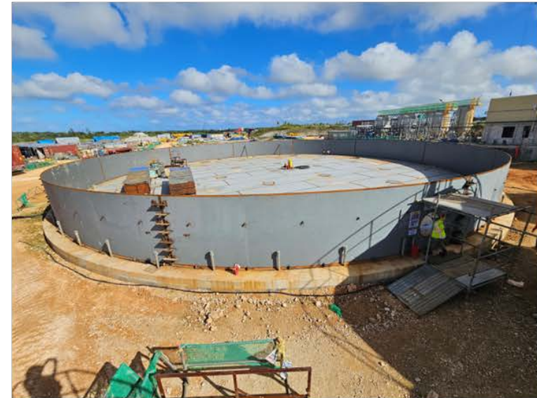
Treated Water Storage Tank B – Restoration of tank walls is in progress.
