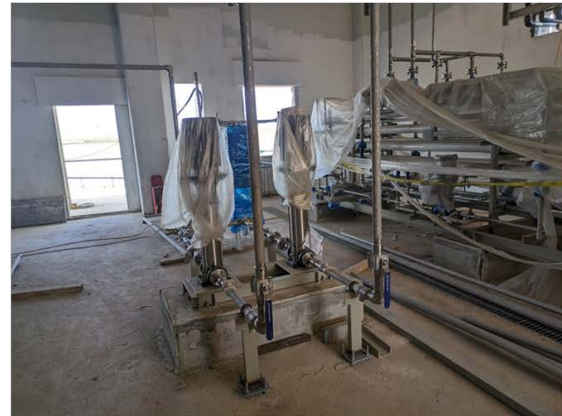
Water Treatment Building – Equipment installation and setup is ongoing
