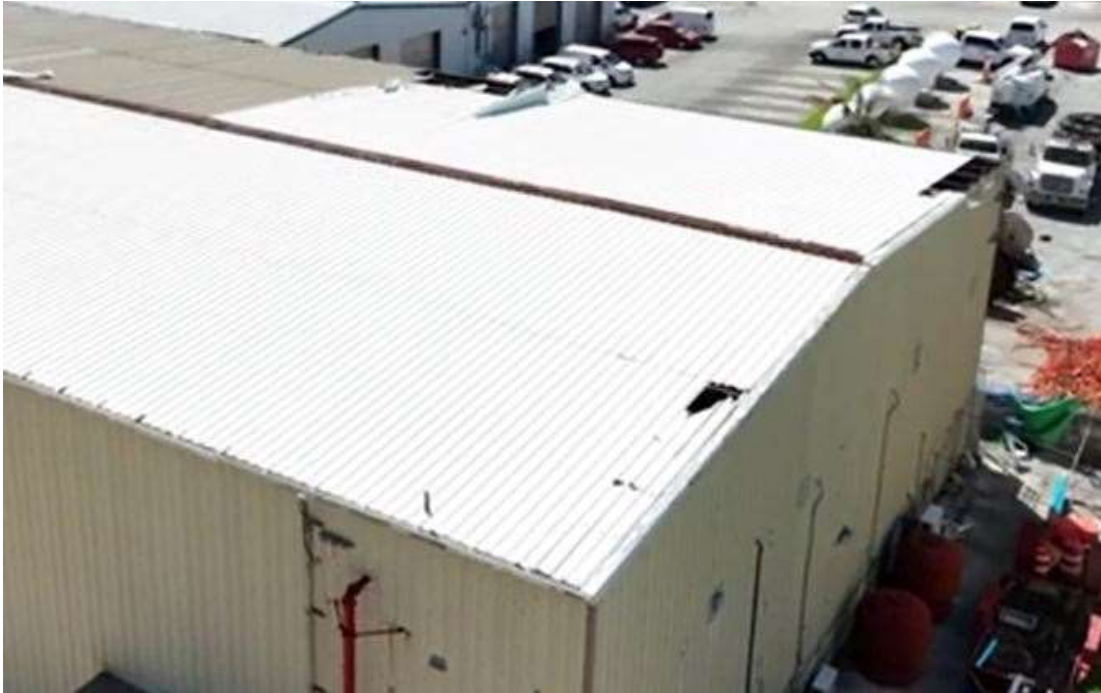
ITEMS 2, 3 & 4– DAMAGED ROOFING AND FLASHING (RIGHT SIDE OF WAREHOUSE)
