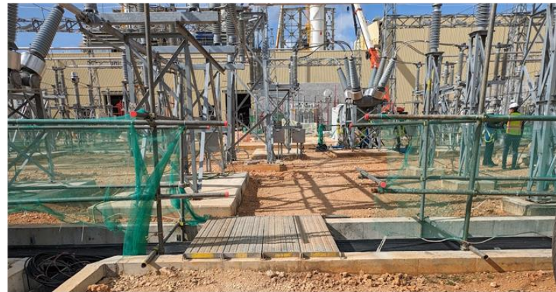
Switchyard Building – Floor is in place. Control room equipment is being set in place
