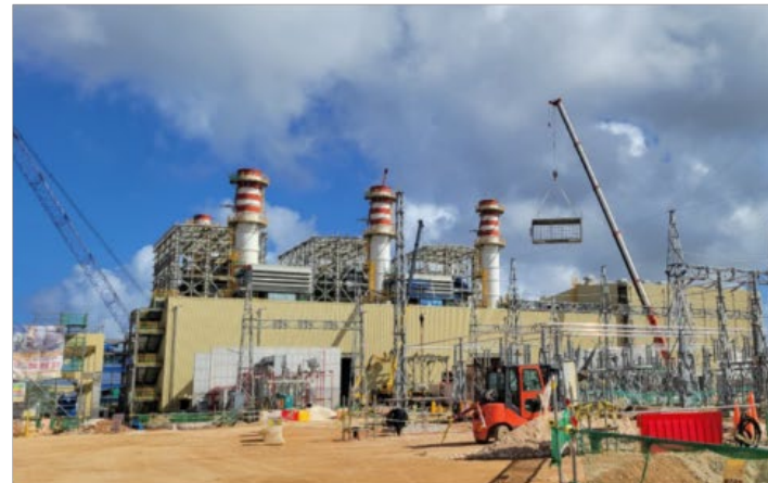
GTG Building – Air intake and piping installation is in progress
