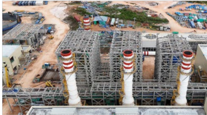
HRSG 1-3: Steel Structure & Drum Installation Work is ongoing
