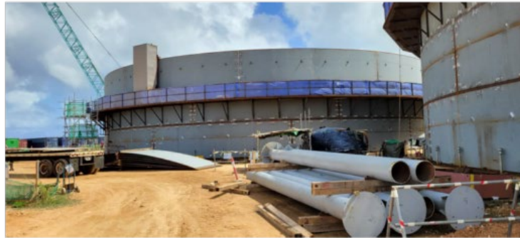
Fire Fighting Tanks – Internal work is ongoing. Preparing for roof installation.
