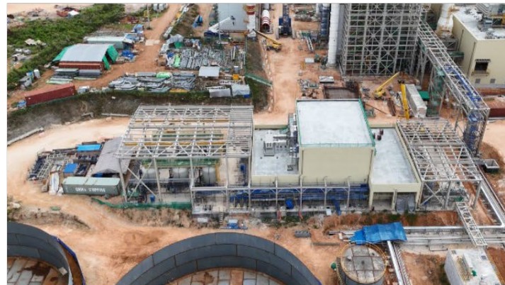
Water Pre-Treatment Area – Installation of pipe supports
