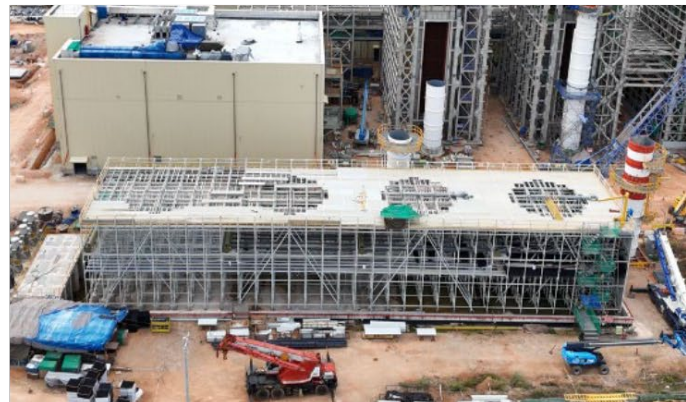
Cooling Tower & Basin – FRP structure assembly is in progress
