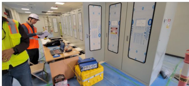
Switchyard Building – Performing Site Acceptance Tests for Control Panel
