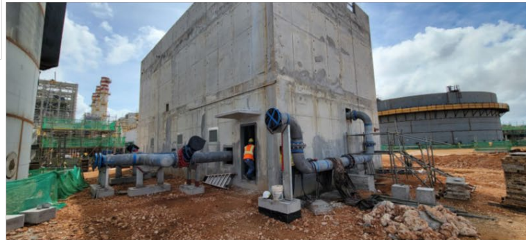
Fire Pump House — External piping towards Firefighting tank is being installed
