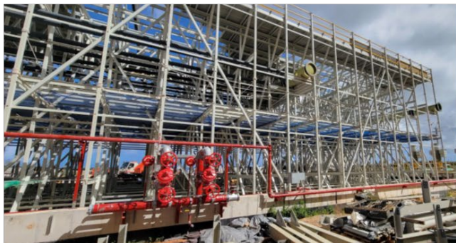
Fire Water Piping installation is ongoing
