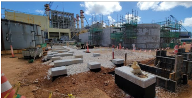
Water Pre-Treatment Area – Installation of pipe supports
