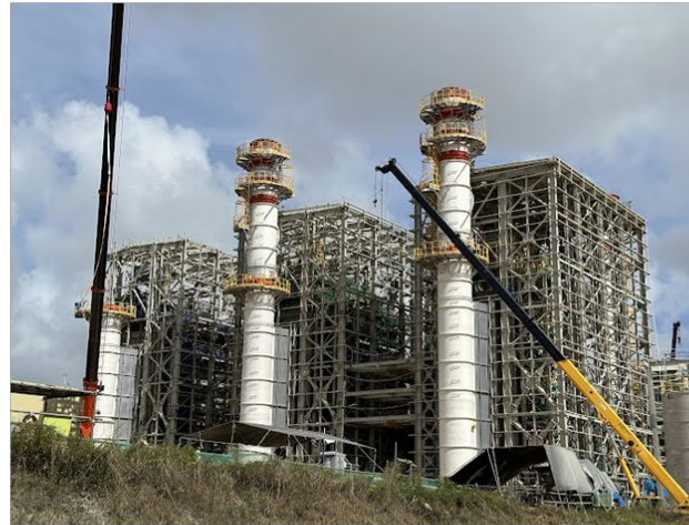
Installation of HRSG 2 outlet stack is completed
