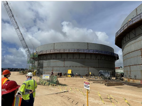
Treated Water Storage Tank A – 4 Courses of Steel Walls are in place
