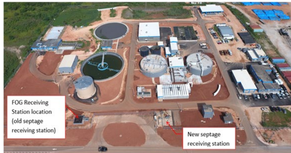
Northern District WWTP FOG Receiving Station
