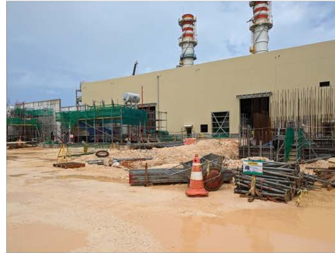
GTG 1-3: Installation of GTG 1-3 ongoing.
