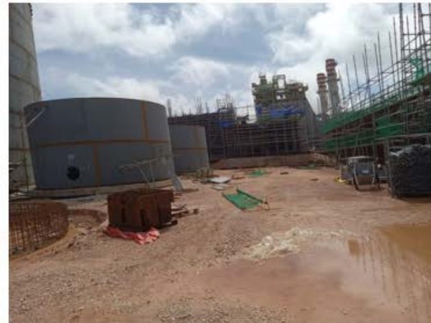
Demineralized Water Tanks – Tanks appear to be undamaged.
