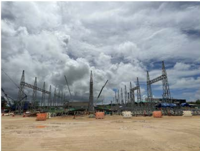
Switchyard – Construction of static line fixtures underway
