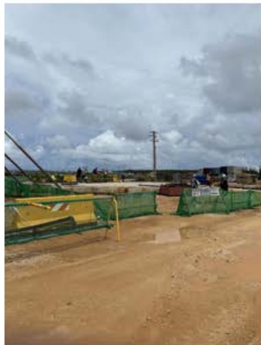
Fire-Water Tank – Demolition completed.
