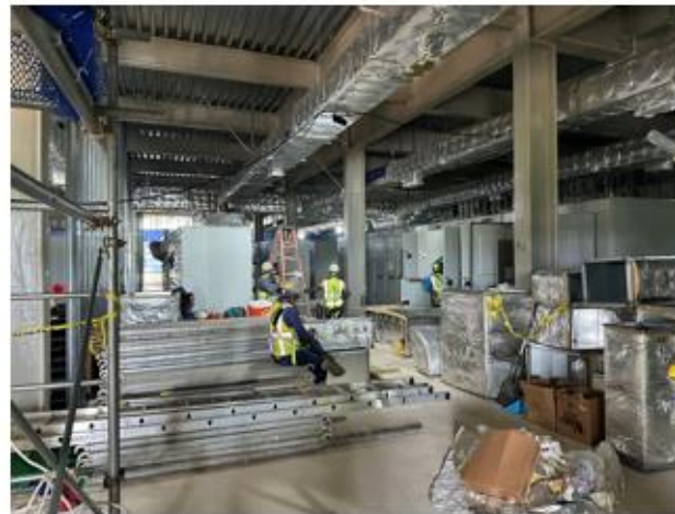
2 nd floor- Switchgear installation ongoing
