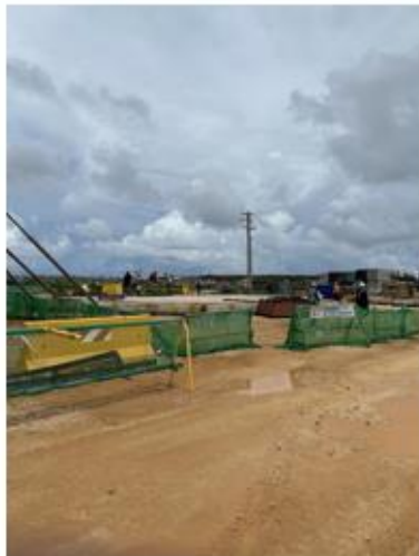
Fire-Water Tank – Demolition completed.
