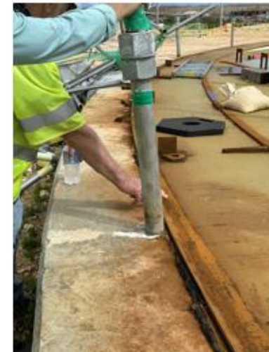
Tank foundations do not require repair
