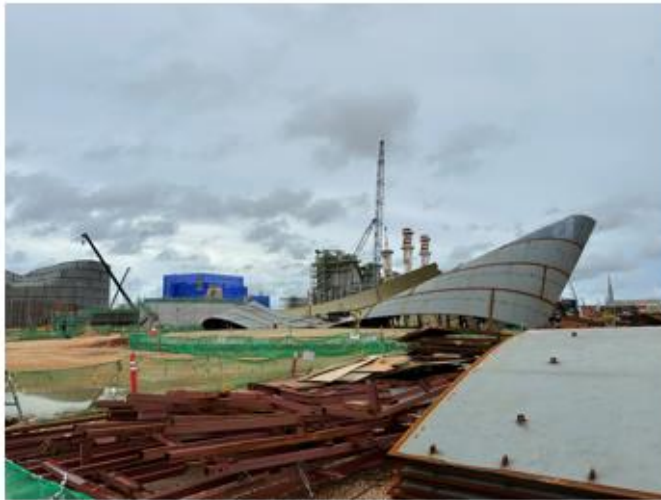
ULSD Storage Tank A – Demolition is ongoing
