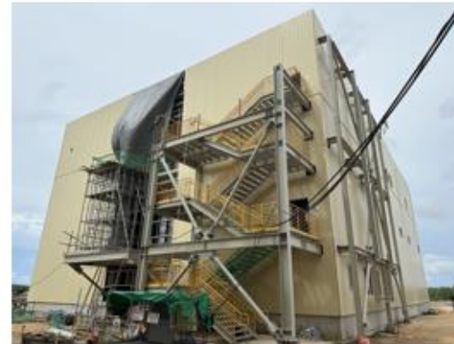
Control & Electrical Building – Exterior side nearly complete
