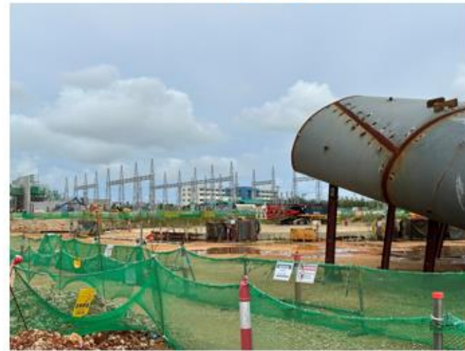
ULSD Storage Tank B – Demolition is ongoing
