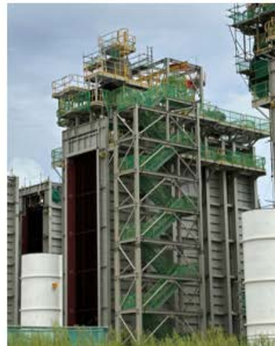
HRSG 1-3: Platform installation and internal welding ongoing
