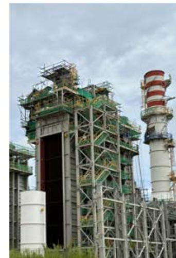
HRSG 1-3: Platform installation and internal welding ongoing
