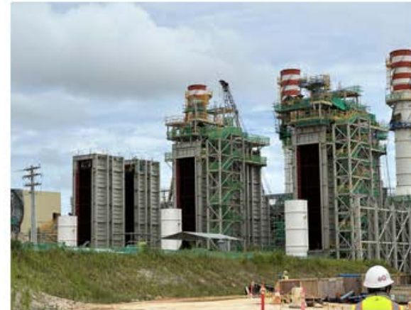
HRSG 1-3: Platform installation and internal welding ongoing
