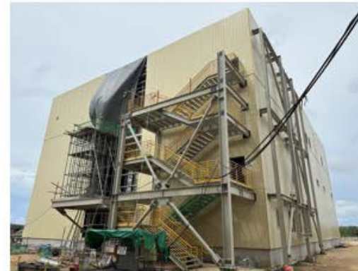
Control & Electrical Building – Exterior side nearly complete
