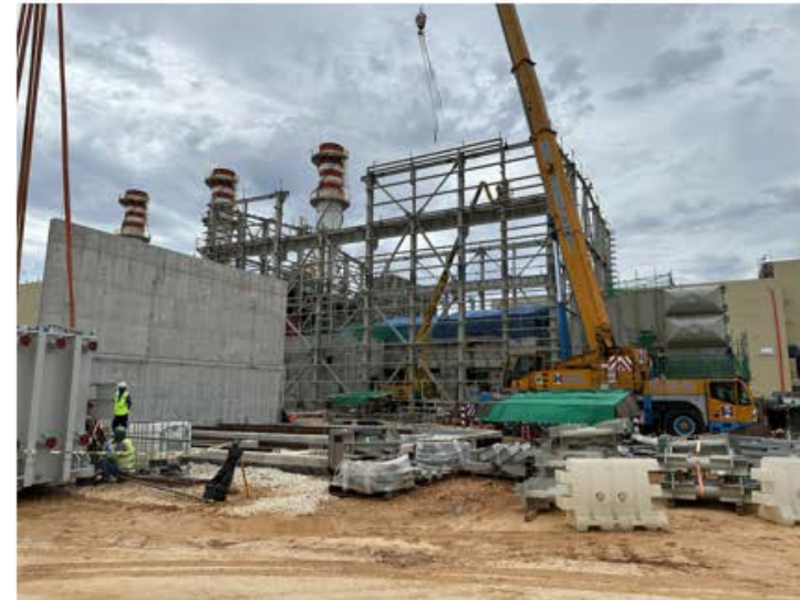
Steam Turbine Generator – Construction of STG building is ongoing
