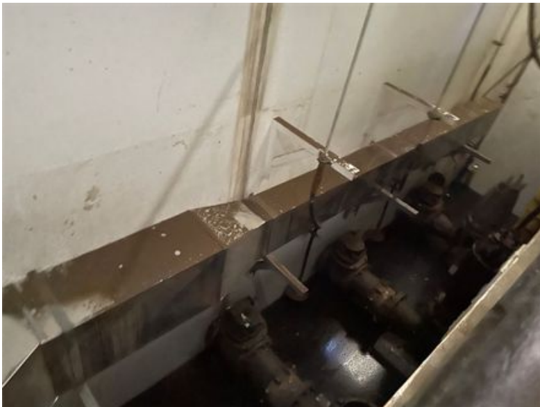
Newly Installed Vent-1
