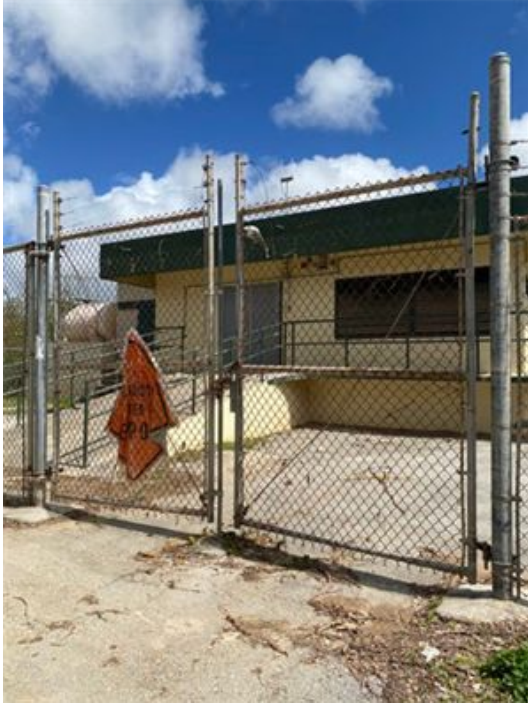
Replace Double Swing Vehicular Gate Fence Fabric and 3- Strand Barbed Wire
