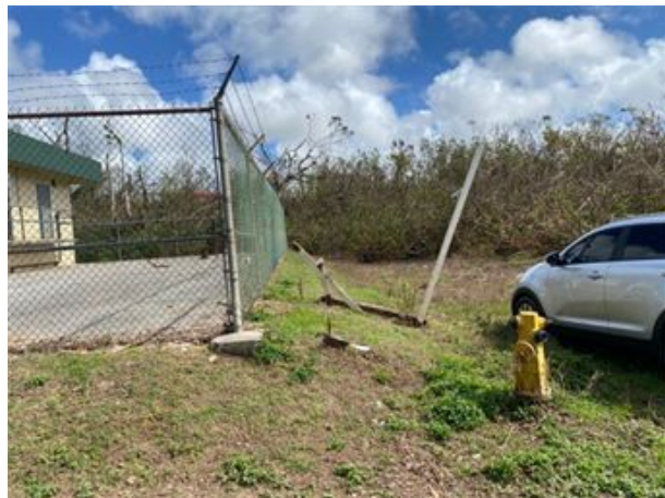
Replace Construction Sign
