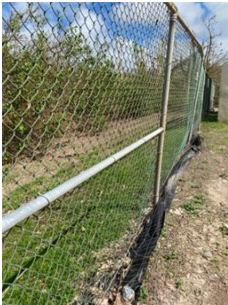
Erect Chain Link Fence Post
