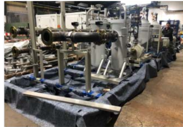
Fuel Oil Treatment System – ULSD Treatment skid manufacturing in progress
