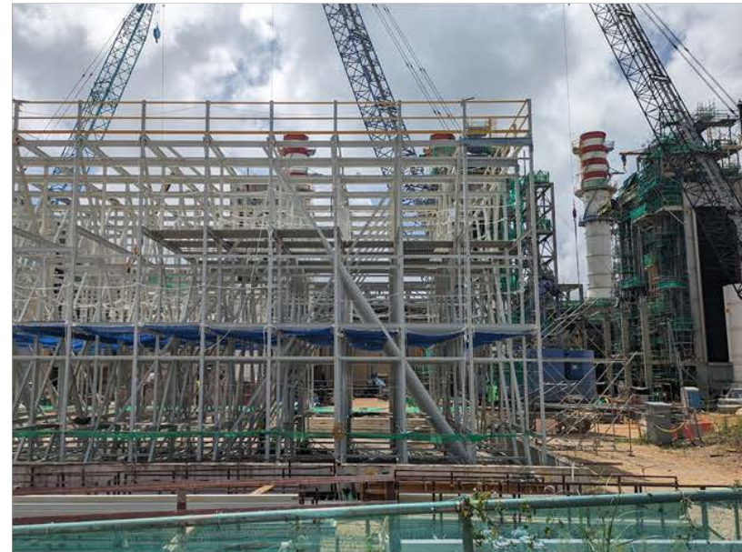
Cooling Tower & Basin – Cooling tower frame installation is nearly complete
