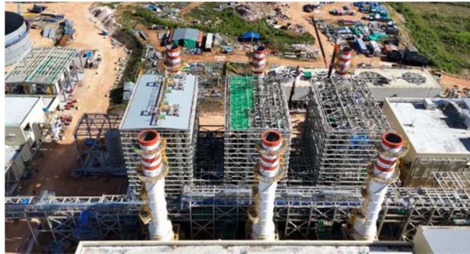
Installation of HRSG 2 outlet stack is completed
