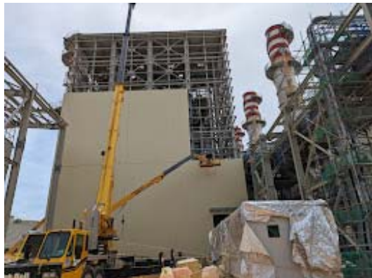
Installation of the HRSG building siding is ongoing
