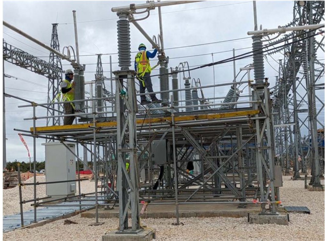
Switchyard – Electrical testing work is ongoing
