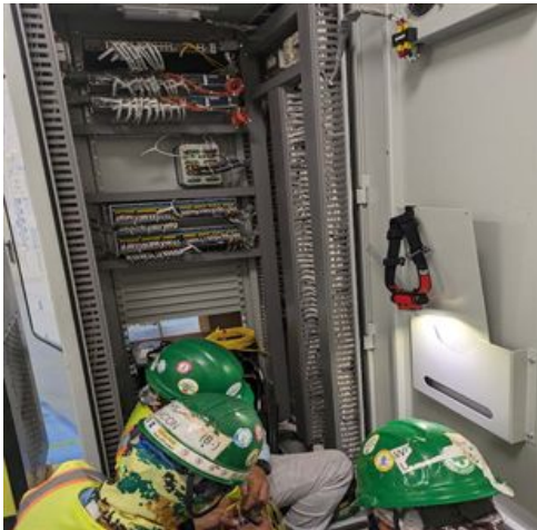
Switchyard Building – Electrical terminations are nearly completed
