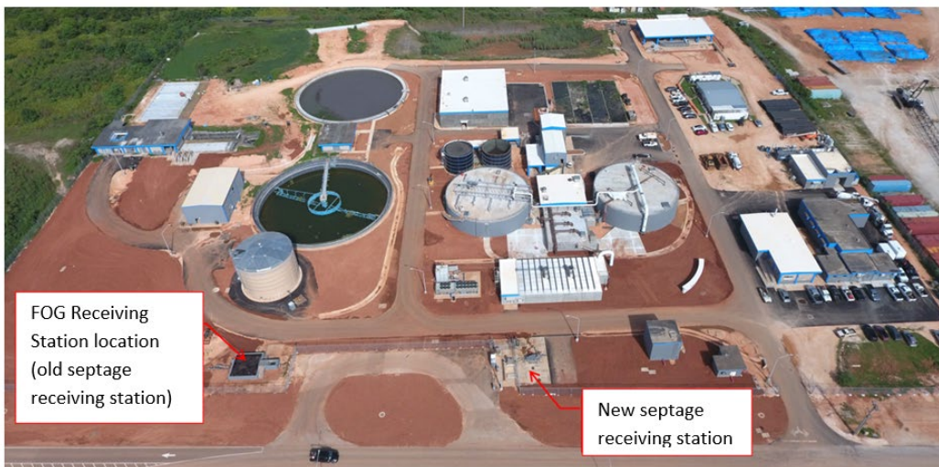
Northern District WWTP FOG Receiving Station
