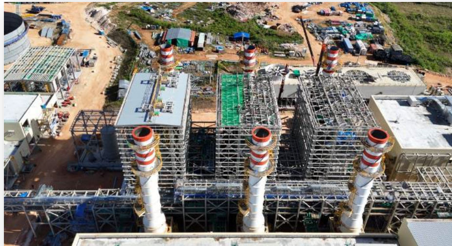
Installation of HRSG 2 outlet stack is completed
