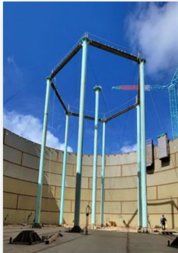
Installation of internal columns are ongoing to prepare for roof installation
