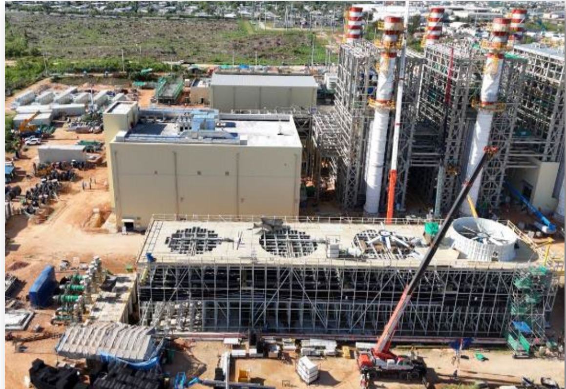
Cooling Tower & Basin – FRP structure assembly is in progress.
