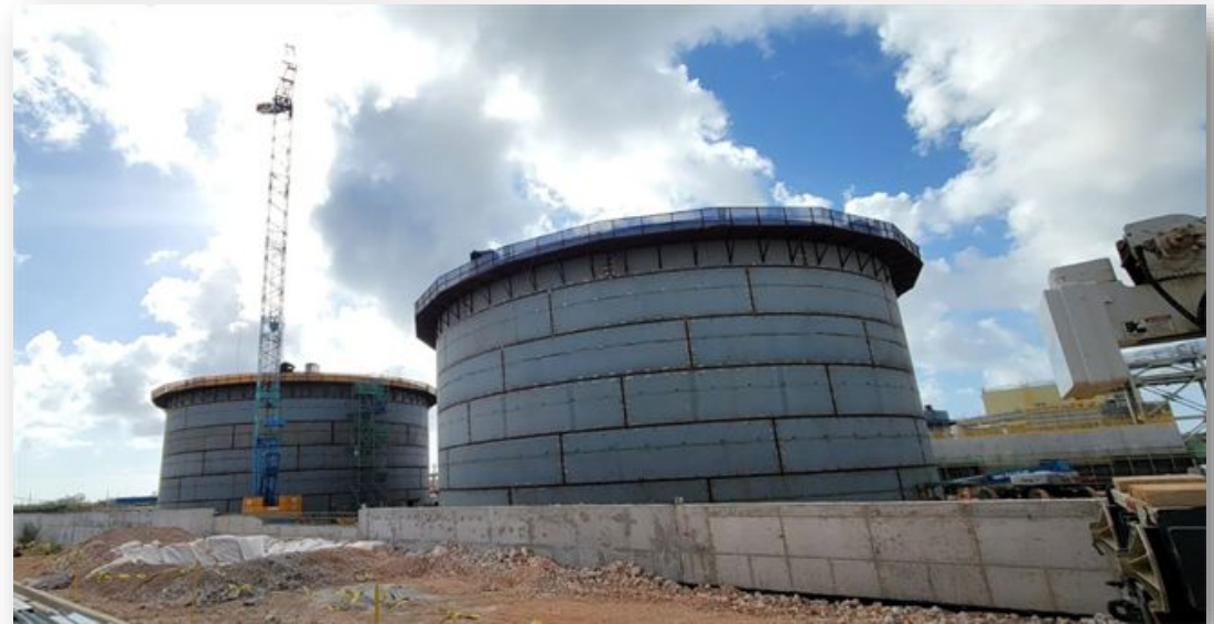
ULSD Storage Tanks – Both Tanks have all 6 courses of steel walls in place
