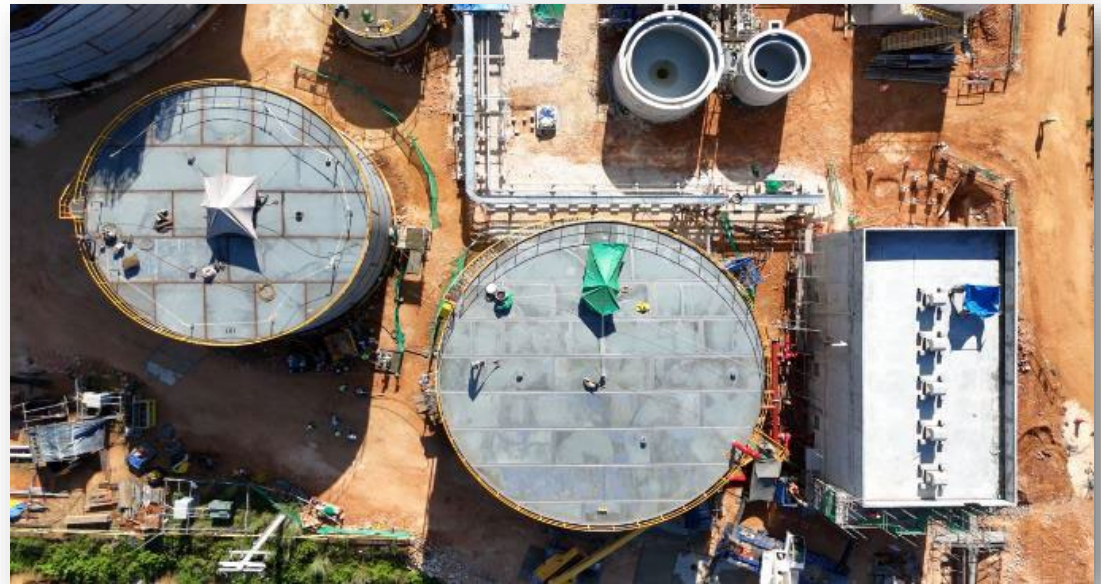
Fire Fighting Tank: Shell plate installation is ongoing
