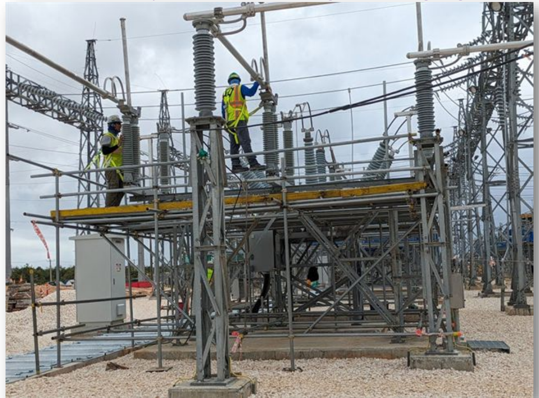
Switchyard – Electrical testing work is ongoing
