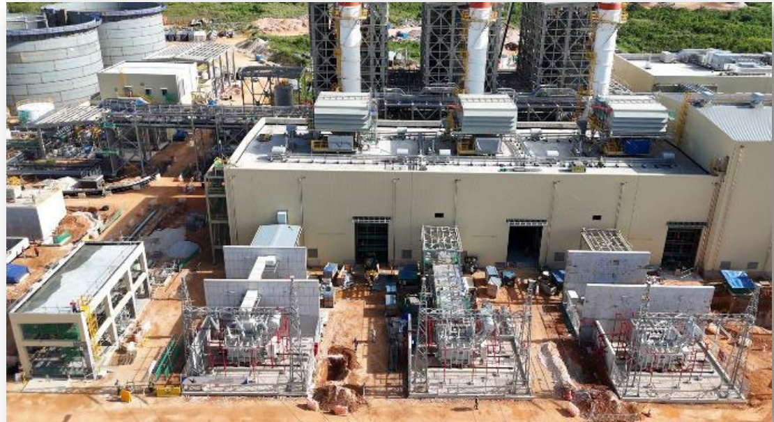
GTG Building – Cable pulling and termination work is ongoing
