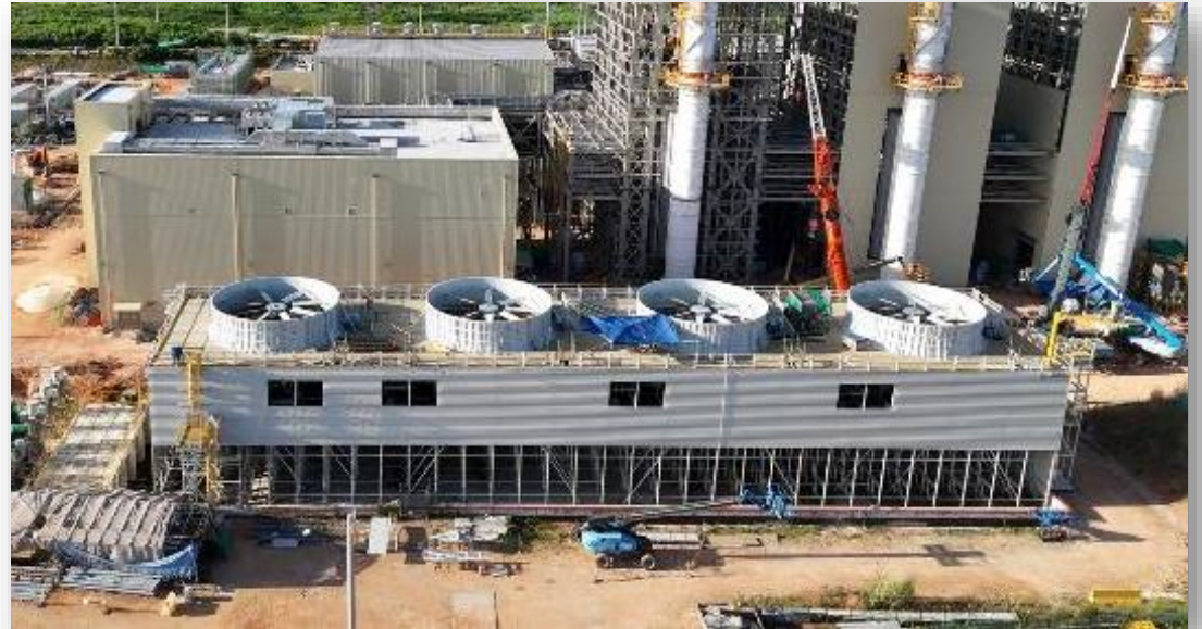
Cooling Tower & Basin – Corrugated panel and Fan Deck installation is ongoing
