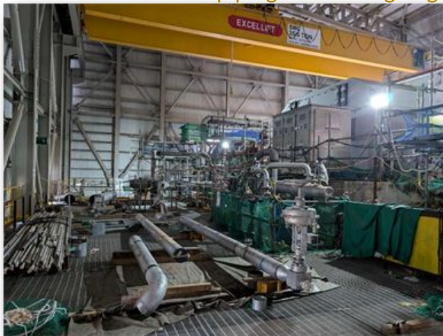
Steam Turbine piping work is ongoing
