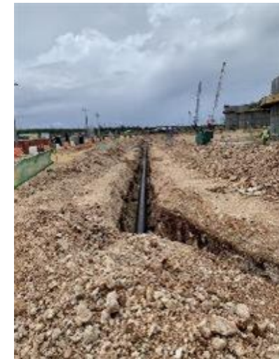
Fire loop installation in progress
