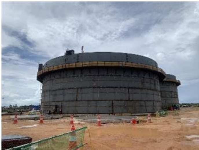
Treated Water Storage Tank 1 – Welding in progress for the 5 th (of 8) row of steel plates
