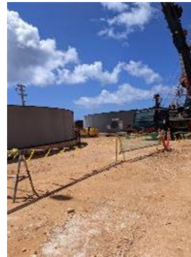
First steel course on fire tank erected
