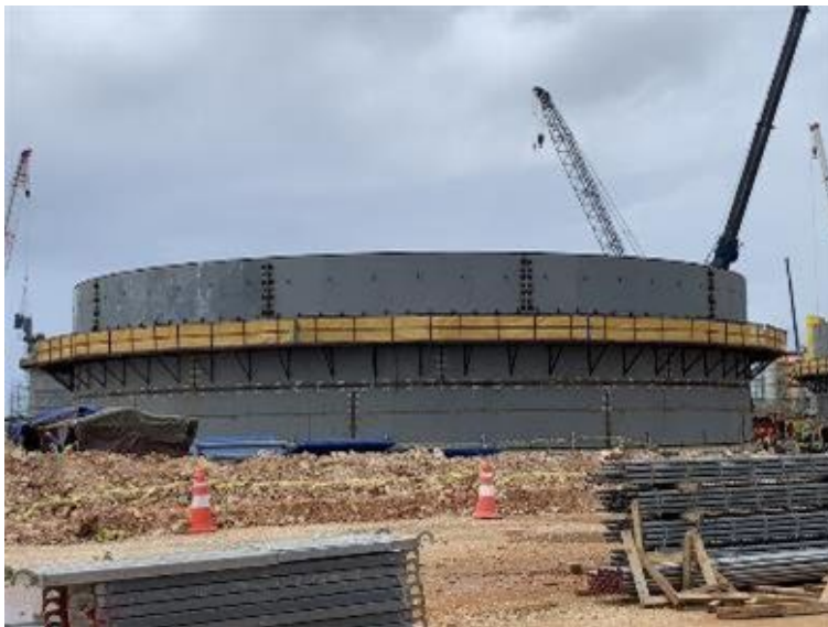
ULSD Storage Tank A— 3 rd Row of Steel Plates Currently Being Welded
