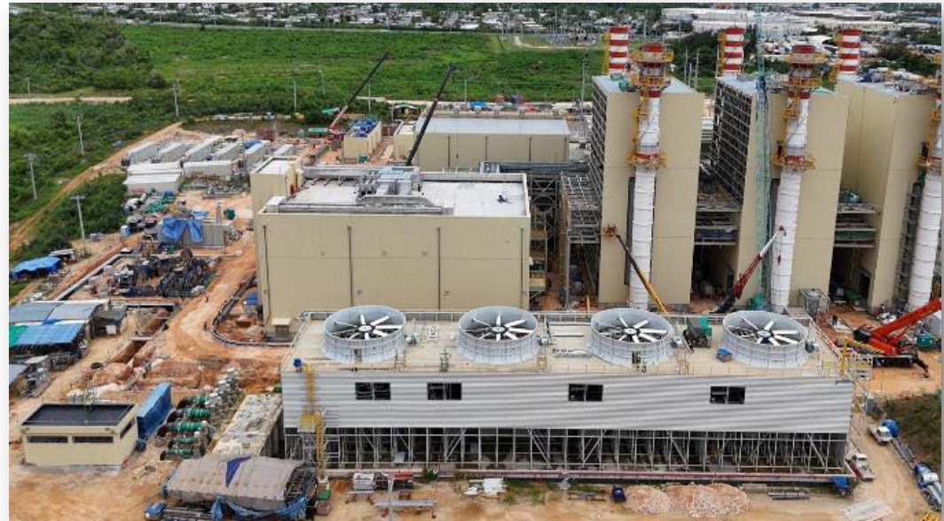
Cooling Tower & Basin – Corrugated panel and Fan Deck installation is ongoing
