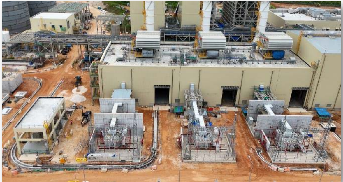
GTG Building – Cable pulling and termination work is ongoing
