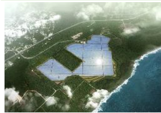
KEPCO Mangilao Solar 60 MW + BESS 32 MW – Ph II
