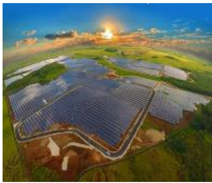
Dandan Solar 25 MW – Ph I
