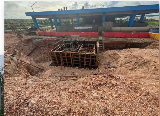
Conduit is being installed towards emergency generator
