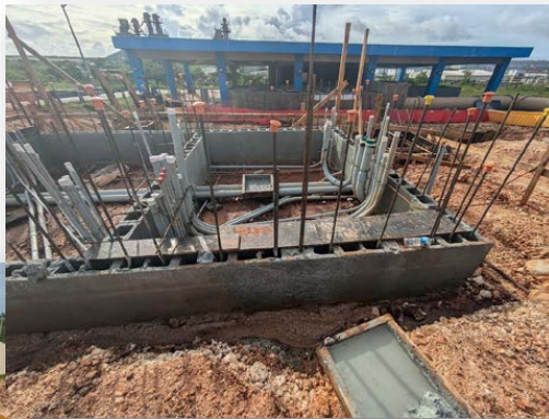
Pipe trench is partially backfilled
