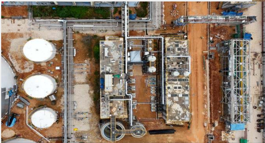
Water Pre-Treatment Building: Pipe fitting is ongoing
