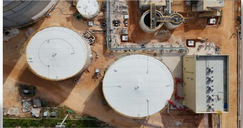
Fire Fighting Tank: U-Ditch installation is in progress.
