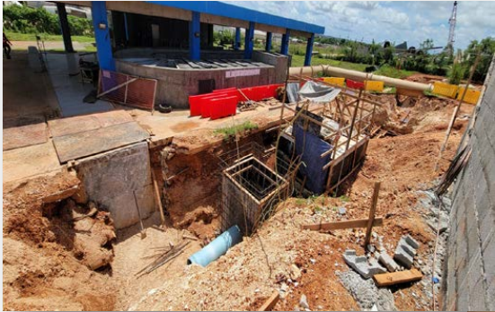
Motorized Valve Pit Forms with Piping
